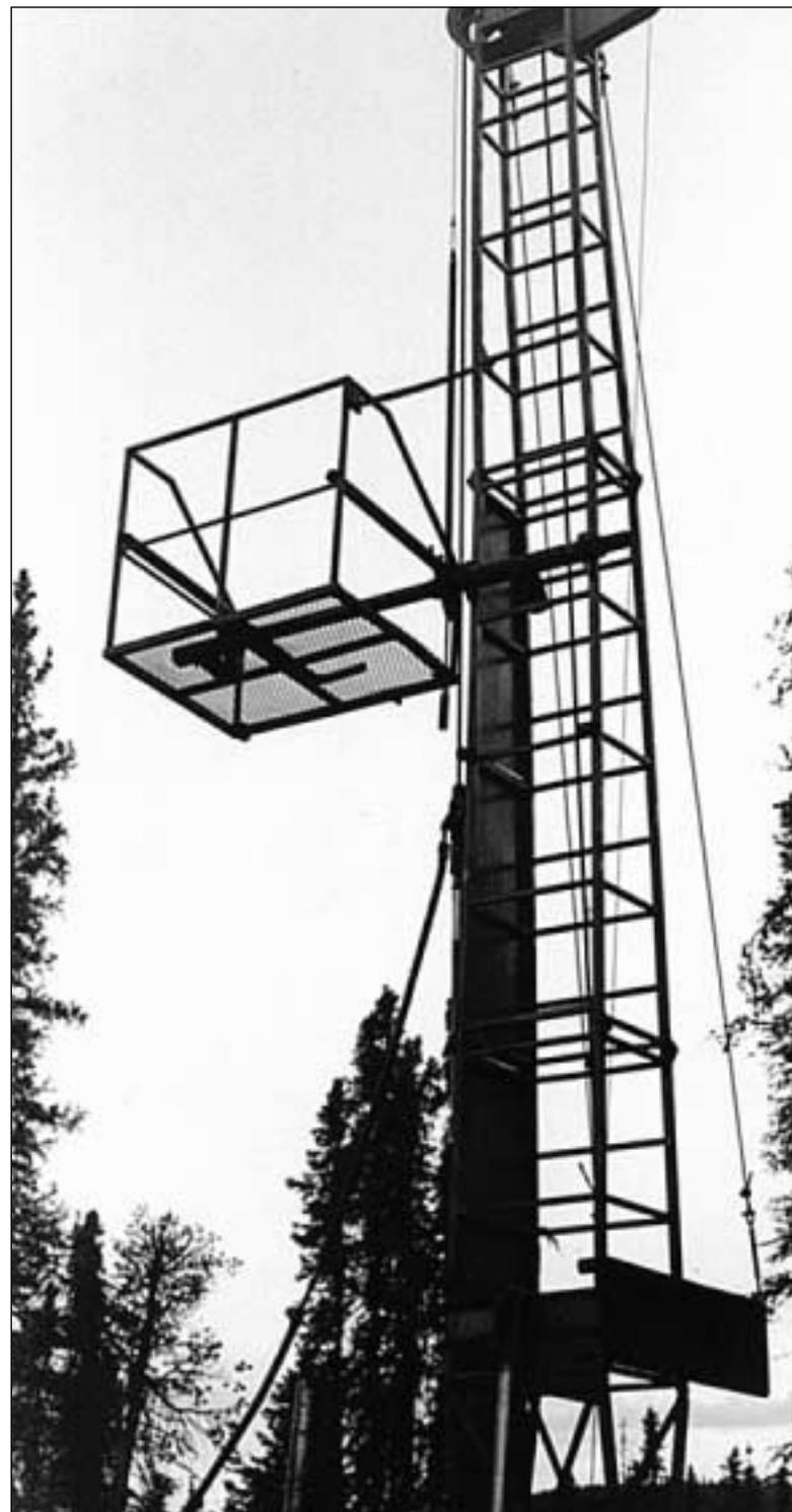
**WORKING DRILL** - A derrick of Caron's diamond drill is seen working at the DEF copper property in 1974. Caron was the first diamond drilling company working in the Yukon to replace tri-poles with derricks.
